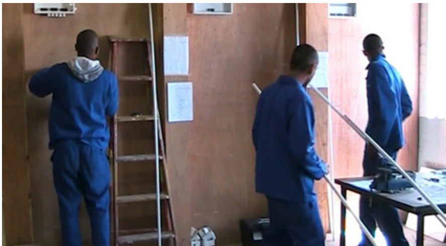
Figure 17: The workshop 'beginning to install wire-ways with an offset'
